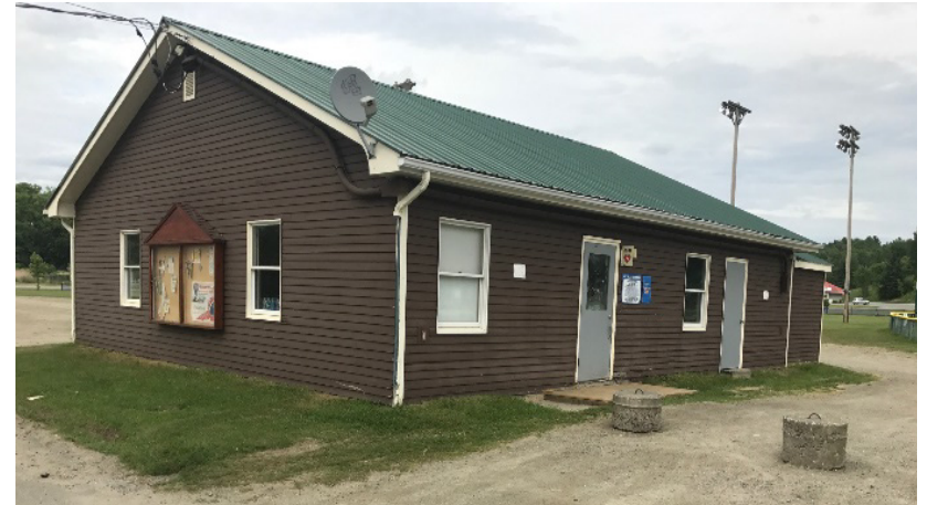
Existing recreation facilities building
